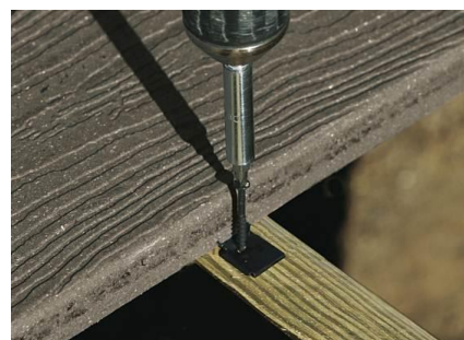
Hidden Fastener Installation to Joist
