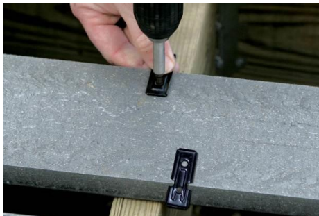
Hidden Fastener Installation to Bottom Surface of Board
